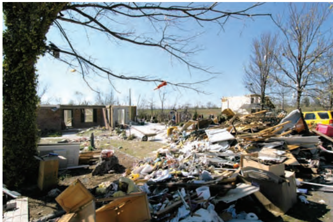
A tornado struck the town of Marmaduke in Green County, Arkansas, on April 2, 2006. Ninety percent of the homes and businesses were affected by storm damage. (FEMA photo by Win Henderson)
