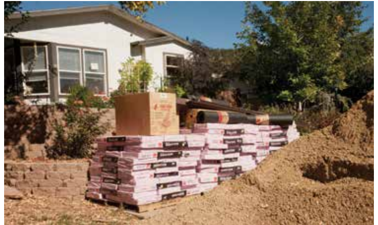
October 7, 2013—Building materials await a contractor who will rebuild a home that was damaged during flooding in the town of Lyon, Colorado. (photo by Patsy Lynch/FEMA)
